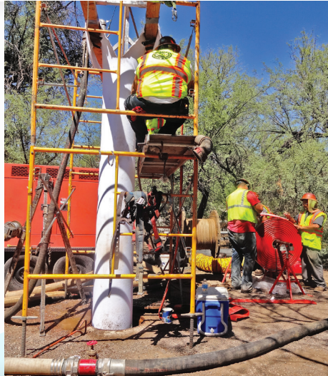
Resin-coated lining is inserted into the manhole.
