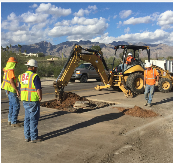
Manhole rehabilitation
