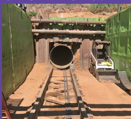
Below – Bore Pit and Tunnel for new piping; Right – Auger used during boring operations.
