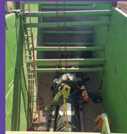
Above – Crews installing pipe into tunnel.
